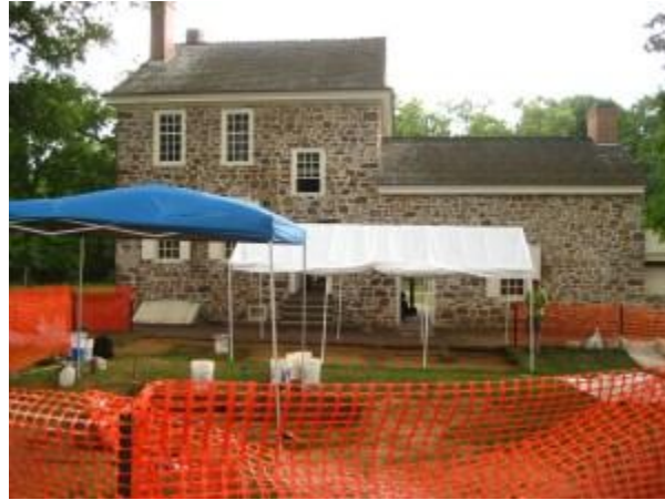
Excavating outside of Washington's Headquarters in 2010.
